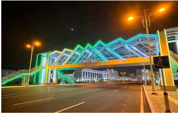
ASHGABAT OVERPASS PROJECT
